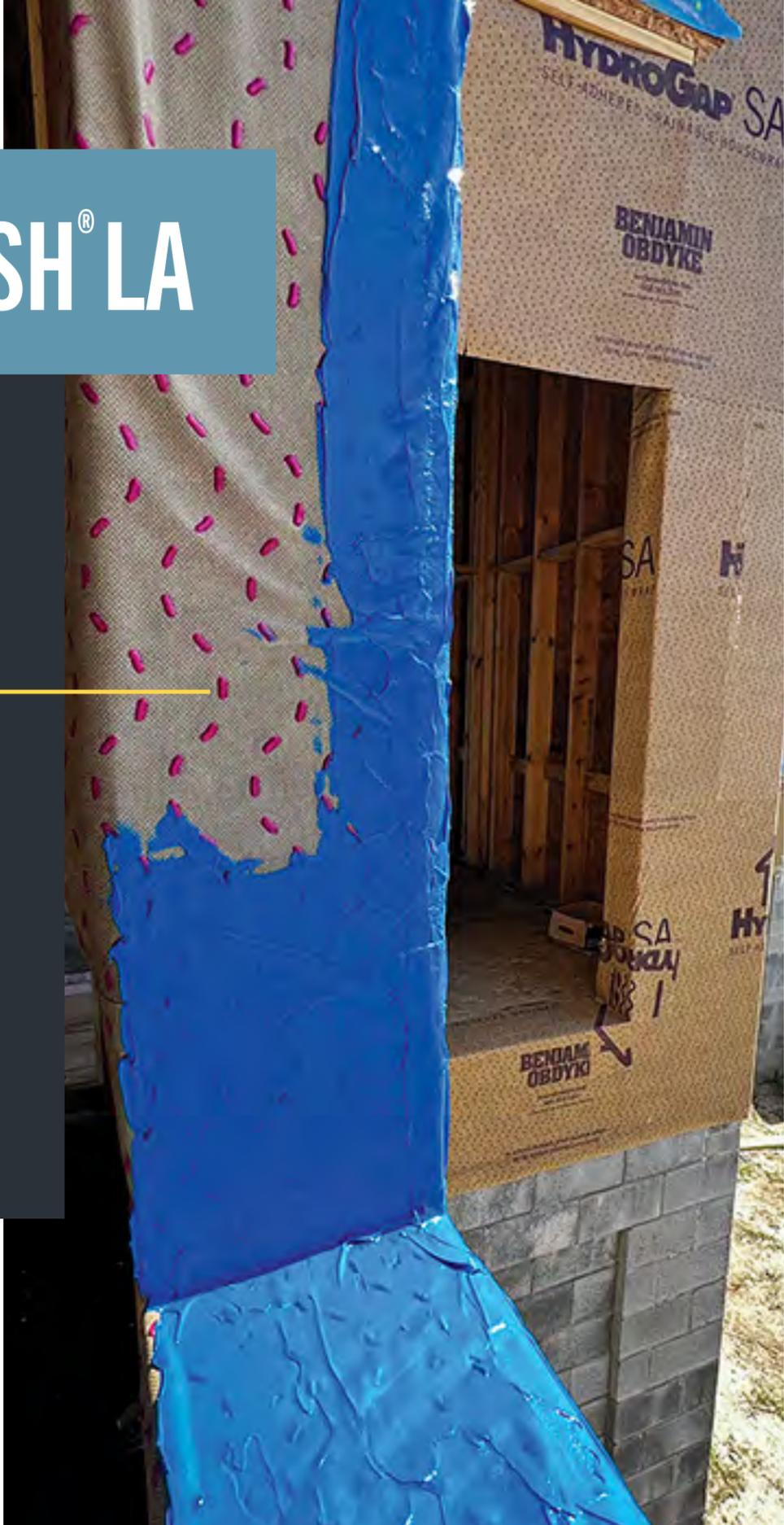
use for challenging details in exterior insulation applications, including geometrically challenging areas
